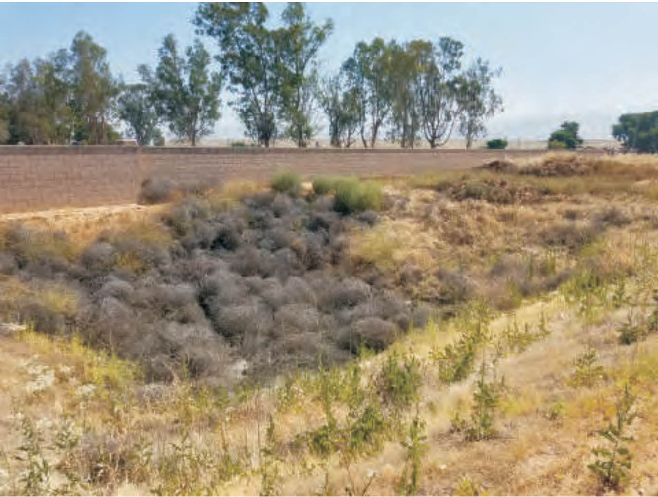
Picture 5. Looking at small drainage sump in north-central area
