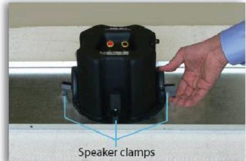
**STEP 9** - Drop the speaker wire down from the empty tile hole in the ceiling and connect it to the speaker. Remove the insulation from the end of the wires. While pushing the plastic tab to open the terminal insert the bare wire into the terminal hole and release the tab. Connect the red wire to the red terminal and the black wire to the black terminal.
