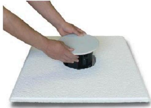
**STEP 7** - Lower the speaker into the hole. The photo shows the speaker being lowered from the side for clarity.
